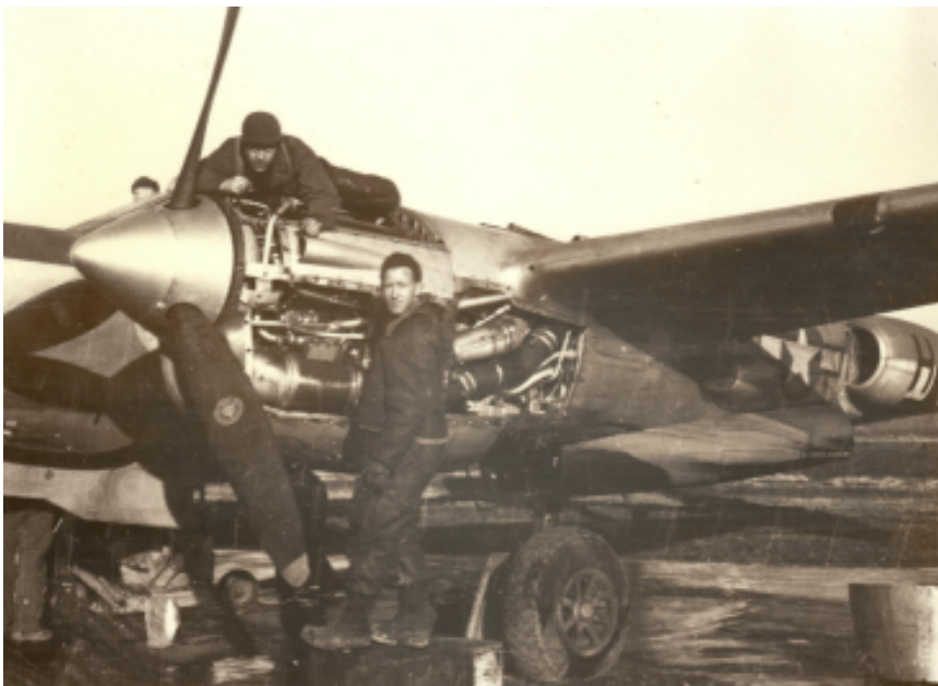
P-38 of the 393rd FS being maintained by the ground crew. Note all the tubing (archives 367 th FG)
