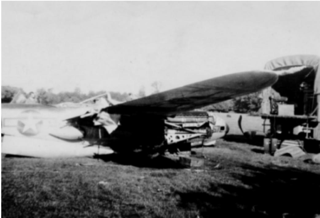
*A truck was parked close to the wreck, certainly to take away the parts that could be used as spare parts for the other Lightnings of the squadron. The part behind the truck are the shell boxes of the canon and the machine guns (Lillian Dillon/archives 367<sup>th</sup> FG)*
